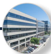
Energy Crossing I 15021 Kay Freeway 240,166 sq. ft.
